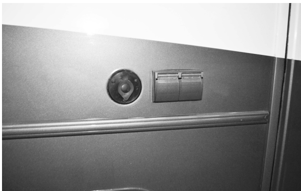
Exterior TV / 12-Volt Connection (Located near entrance door) -Typical View
